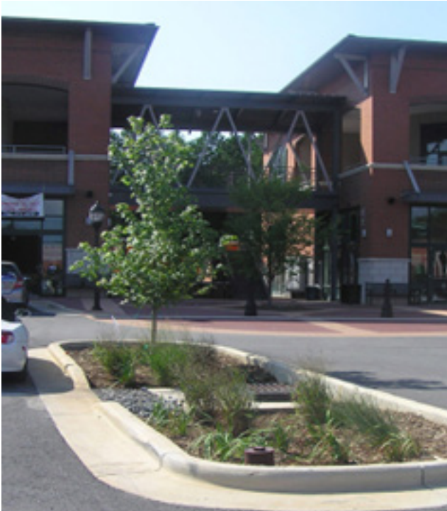
The above photos show the same site at completion and a year later. The parking lot island includes a notched cut that allows parking lot runoff to drain to a stormwater management system that both filters pollutants and infiltrates runoff. (Photo, copyright Randall Arendt, 2015.)
